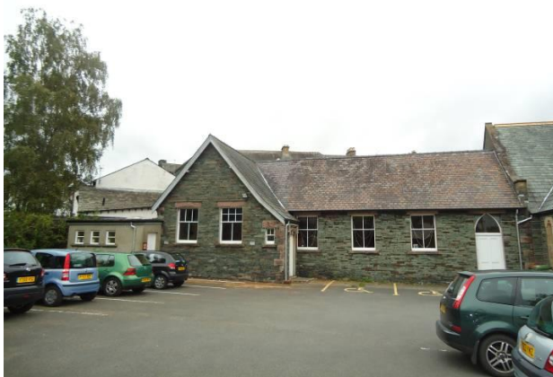
View of rear of church and car park showing area to be sold for development of affordable housing.
